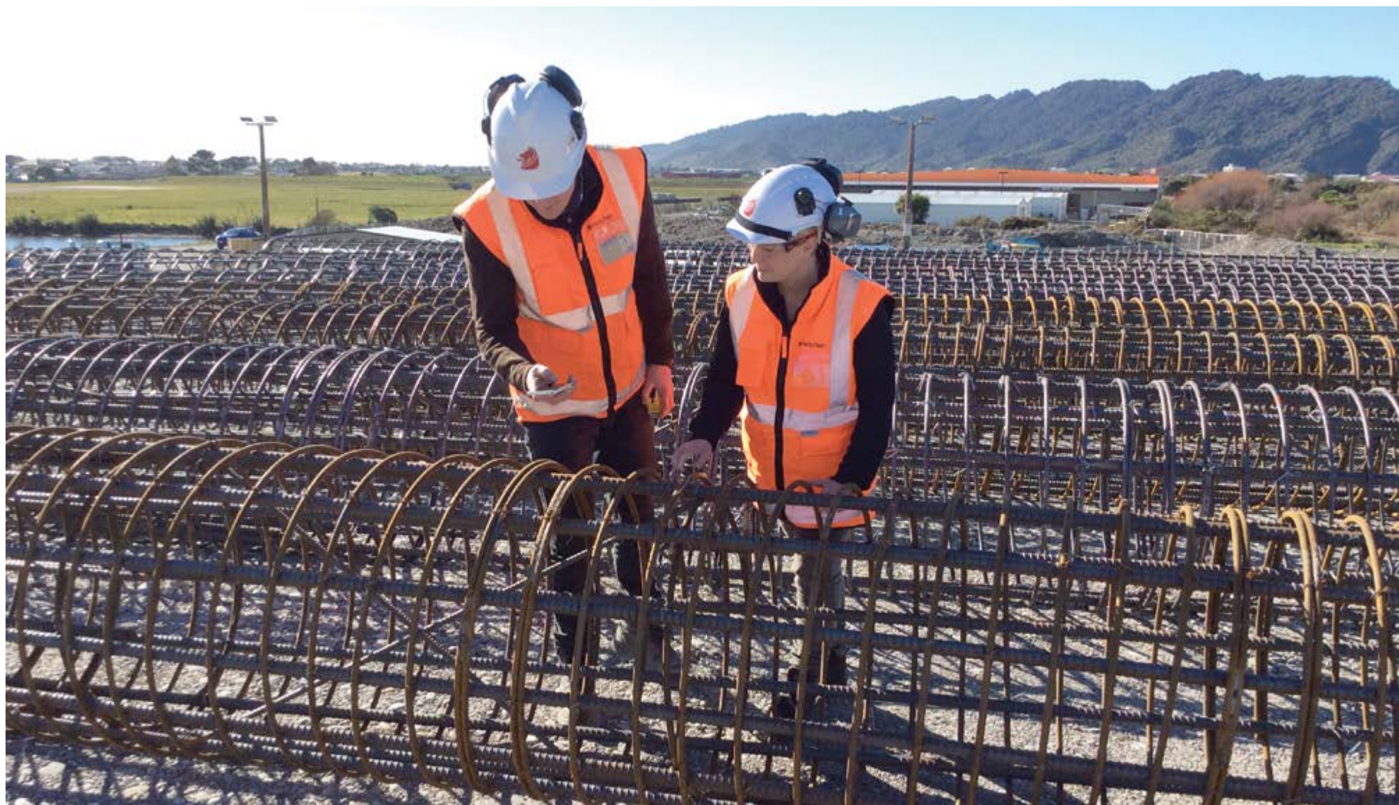
Fletcher Engineer Sam O'Donnell and Health & Safety Advisor Bernadette Olsen check steel cages lined up on the new Grey Health facilities site.
