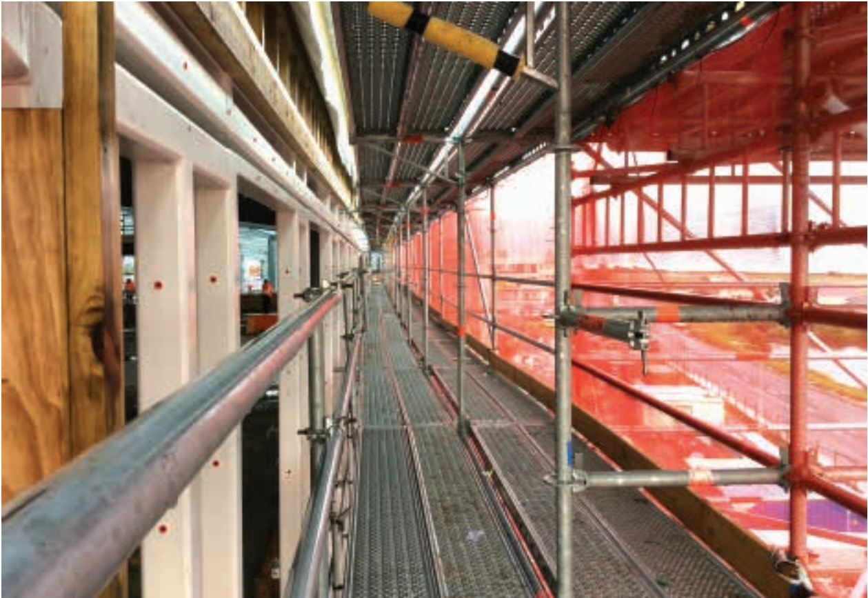
Scaffolding allows workers to access the outside of the new Grey health facility.
