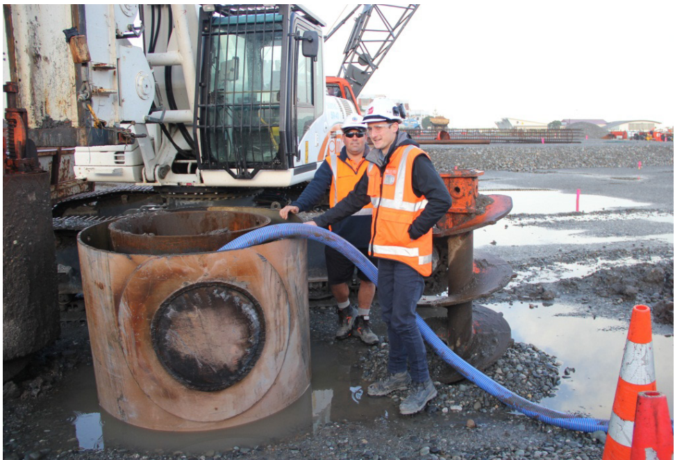
March Construction foreman Steve Williams and Fletcher Construction Project Engineer Sam O'Donnell with the casing for the first Grey Base Hospital pile.
