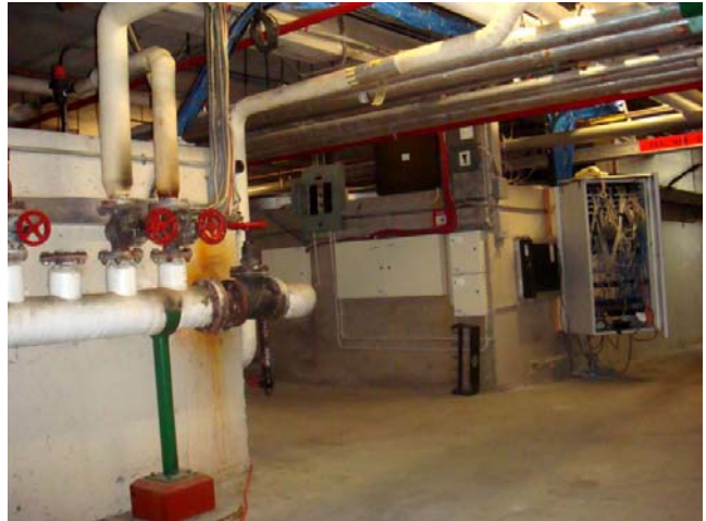
Main service duct. IT and electrical services are at risk in the case of a pipe leak.
