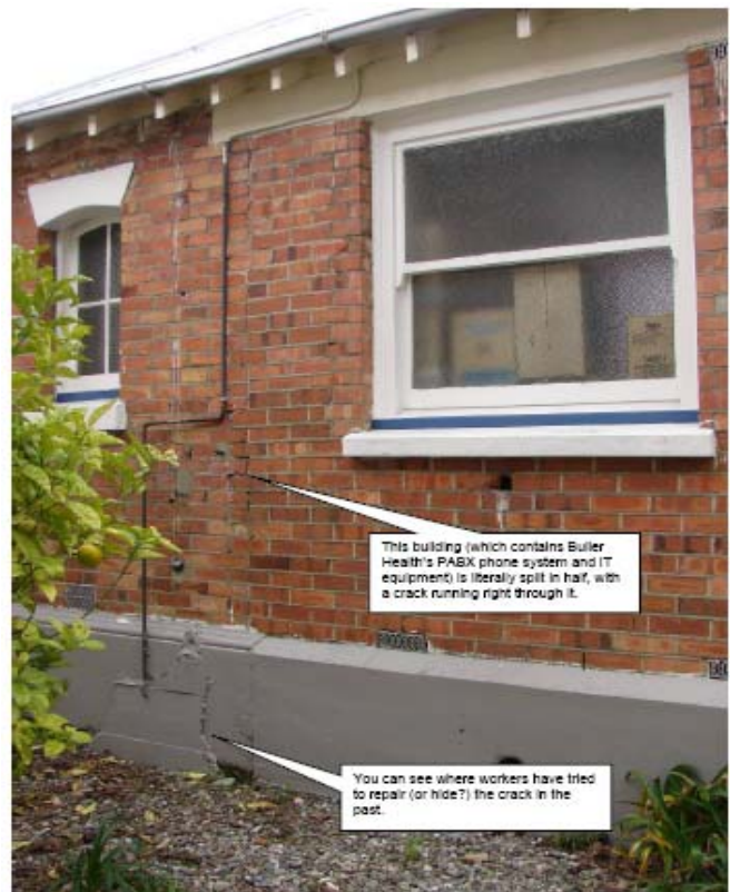
An example of a building with severe structural flaws (PABX / IT Building)
