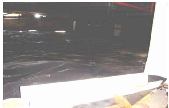
Black polythene on the basement floor is in place in order to encapsulate asbestos.
